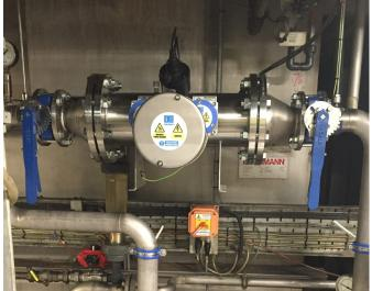
Correctly sized UV systems can aldo be used to de-chlorinate or de-ozonate process water.
